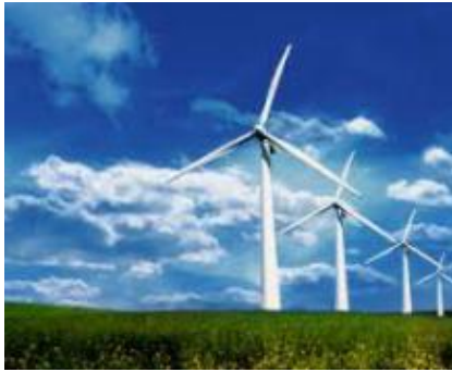
Wind power fans
